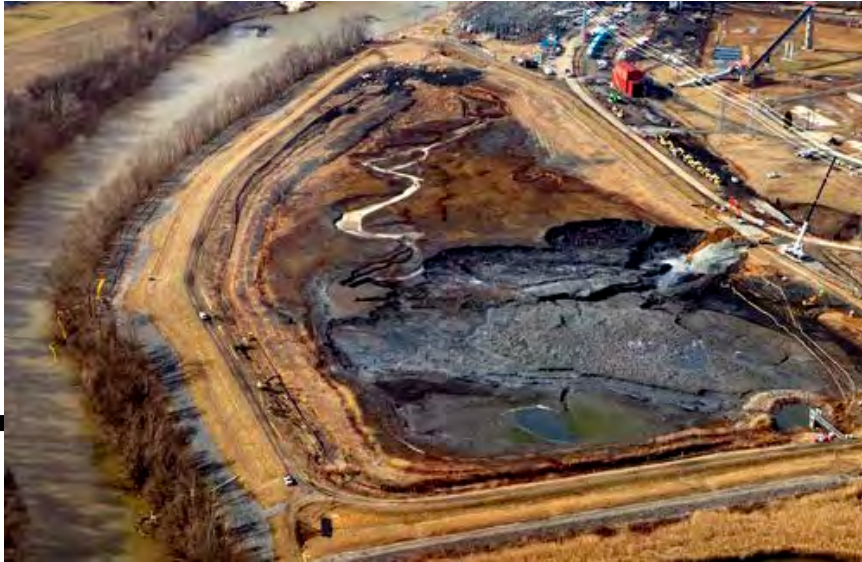
Failure in the wet stack's dike
